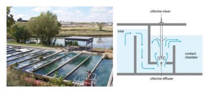
Figure 24 – Chlorination Basin (left), Chlorine dosing and mixer (right)
